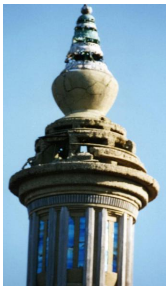
close-up of finial on smoke stack minaret of power house pictured above
